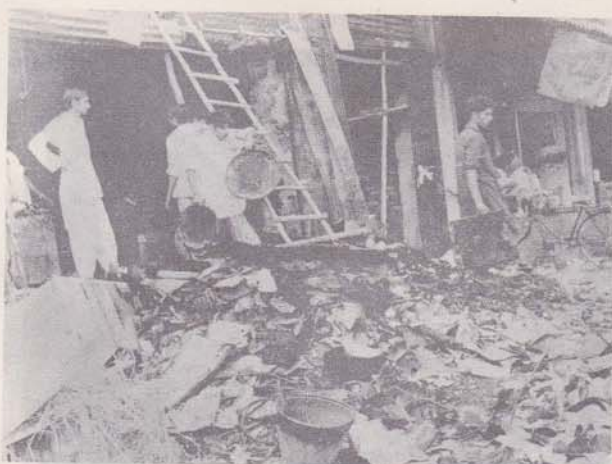
Ahmadi houses looted and demolished
